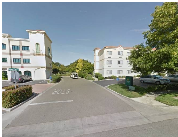
30. View of adjoining property to west across Research Park Drive, La Quinta Inn & Suites.
