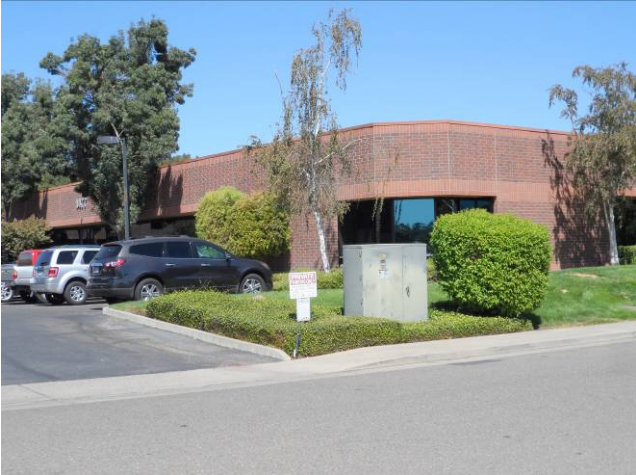
7. View northeast of Building 1477 west and south façades.
