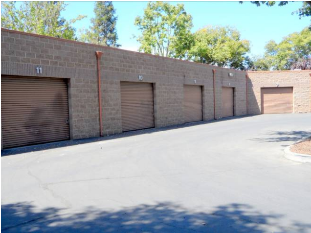
10. View west of Building 1921 east façade.
