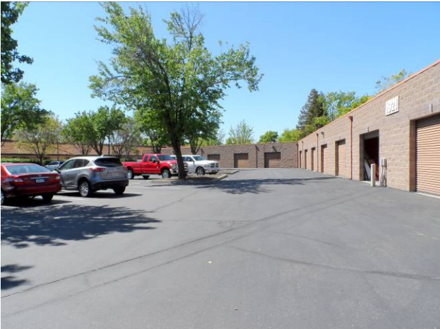
9. View west along Building 1921 southeast façade.
