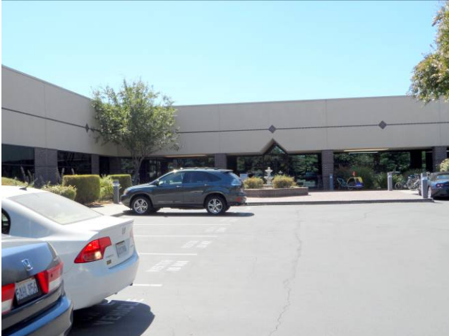
8. View southwest of Building 1850 northeast façade.
